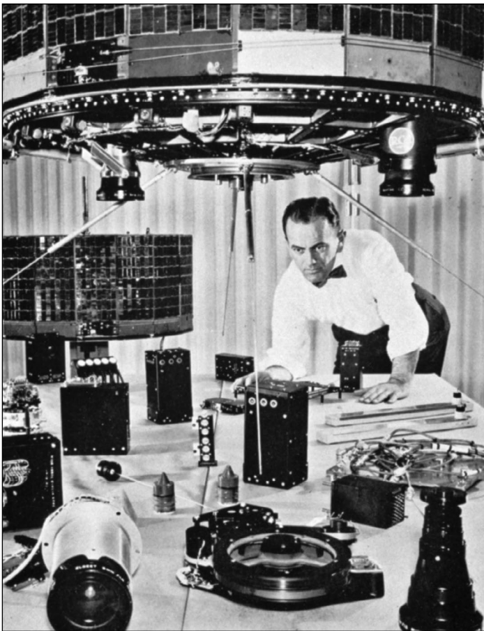
Figure 4 - TIROS instrumentation, cameras in the foreground with the tape recorder between them
